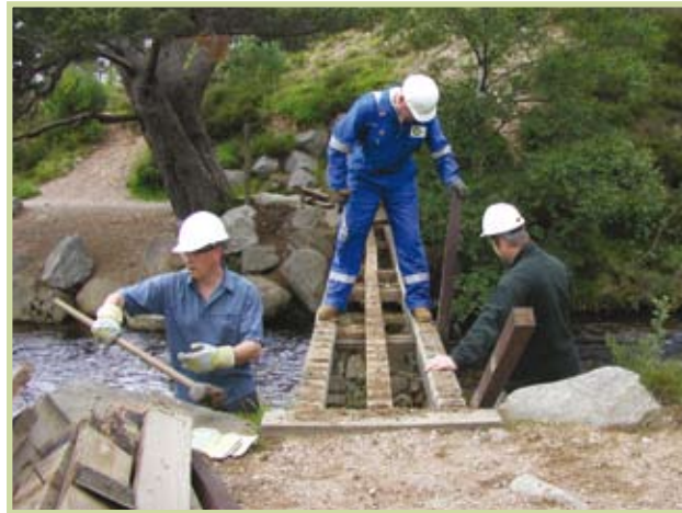
FCS - Bridge building at FCS Glenmore
